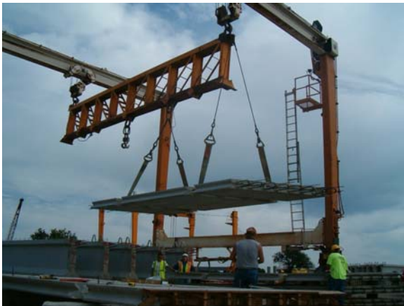
Figure 21 – Deck Panel Stockpiling
