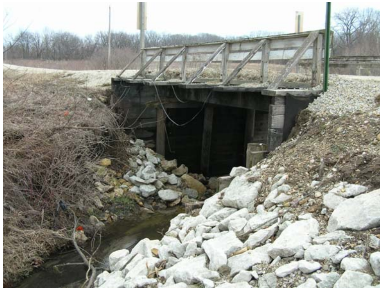
Figure 61 - Existing timber bridge carrying secondary road over small stream
