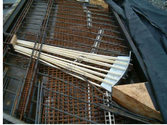
Figure 20 – End Panel Bottom Reinforcing Only
