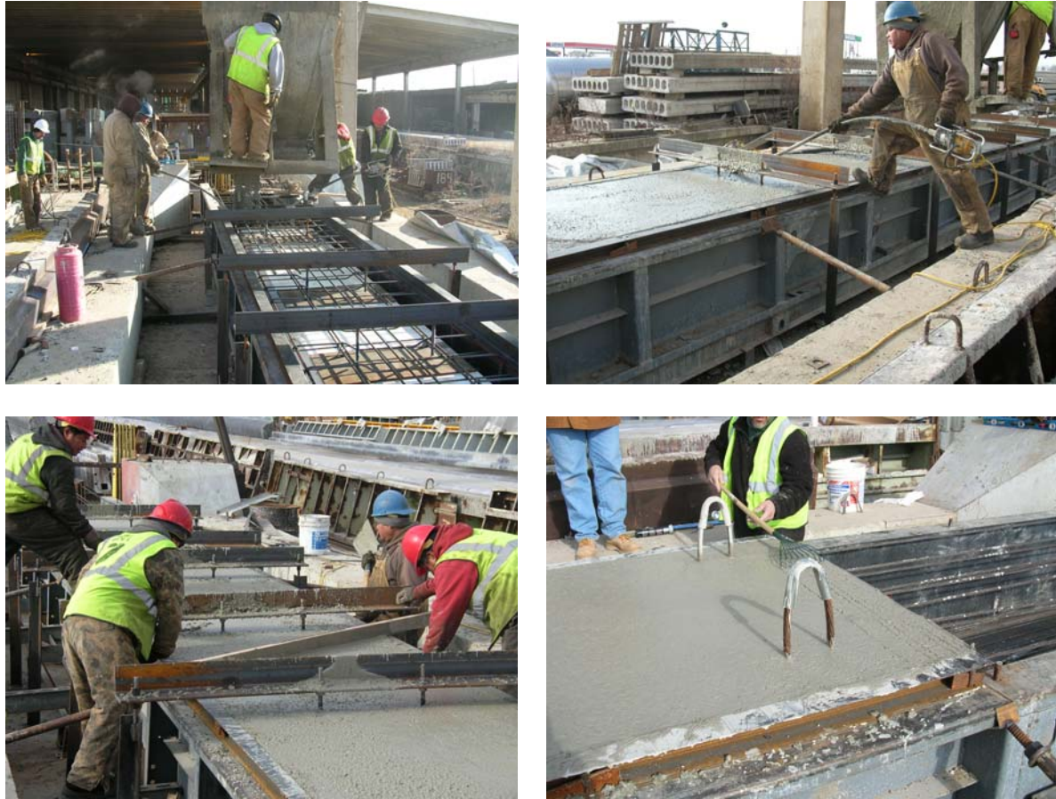
Figure 66 - Casting of the box beams
