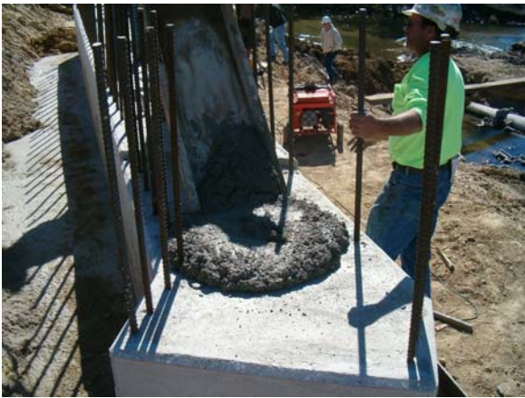
Figure 27 – Filling Abutment Blockout
