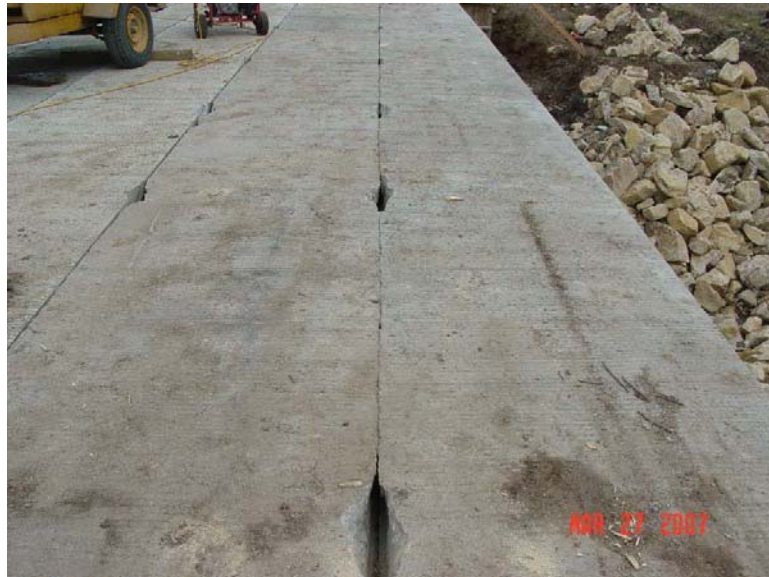
Figure 72 - Longitudinal joint showing contractor's increased width along span
