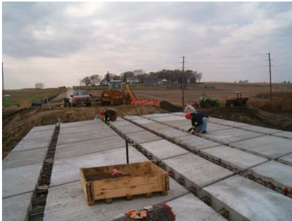
Figure 38 – Leveling Device Installation
