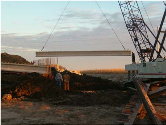
Figure 31 – PPC Beam Setting
