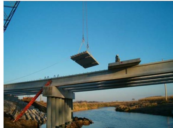
Figure 36 – Deck Panel Erection
