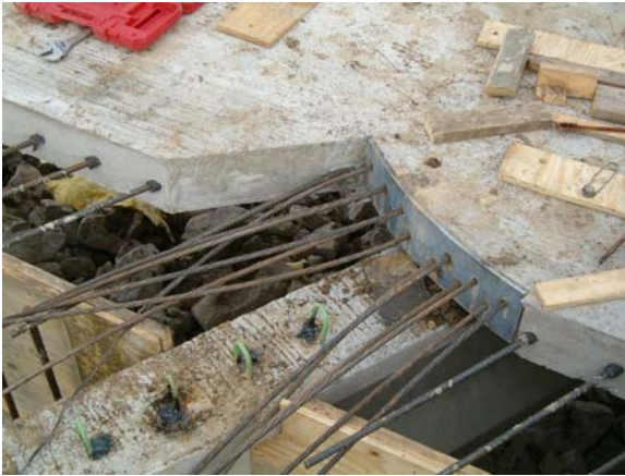
Figure 42 – PT Strand Anchorage
