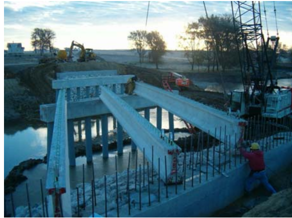
Figure 32 – PPC Beam Setting
