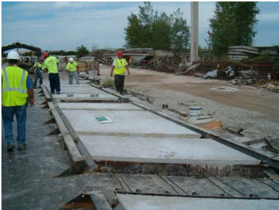
Figure 15 – Panel Form Release
