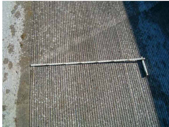
Figure 51 – Longitudinal Grooving
