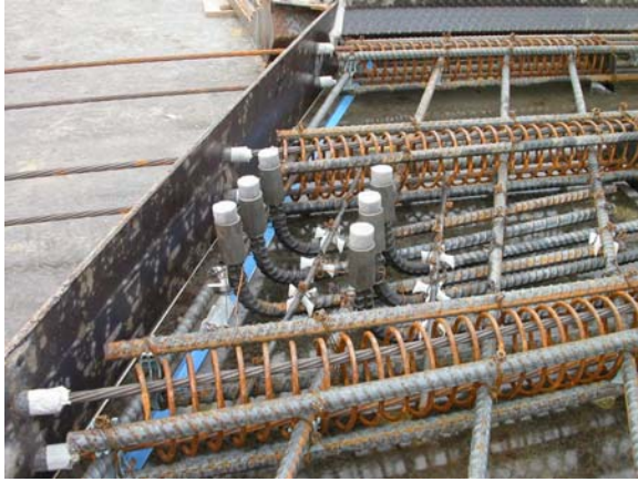
Figure 19 – Mechanical Splicers
