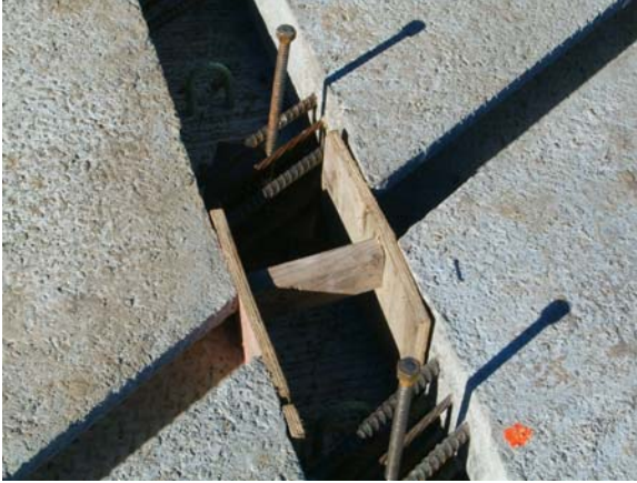
Figure 40 – Transverse Joint Form
