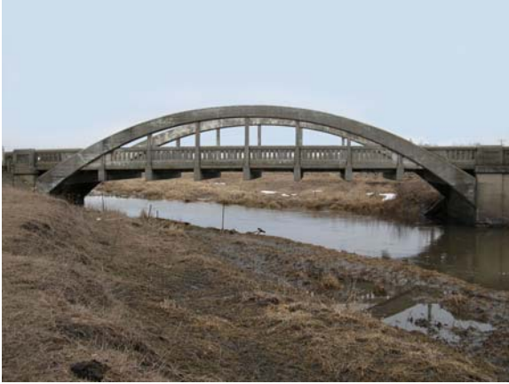
Figure 1 - Marsh Arch Bridge
