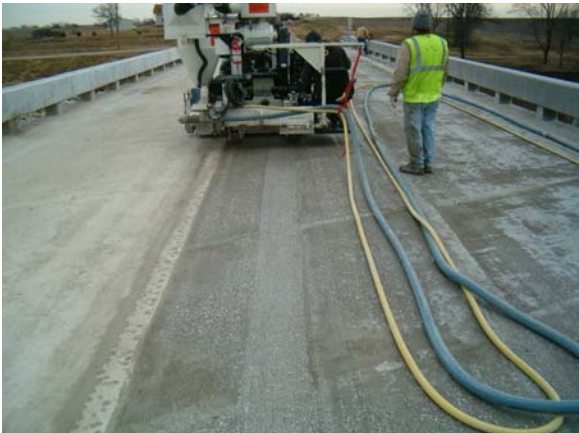
Figure 50 – Longitudinal Grooving
