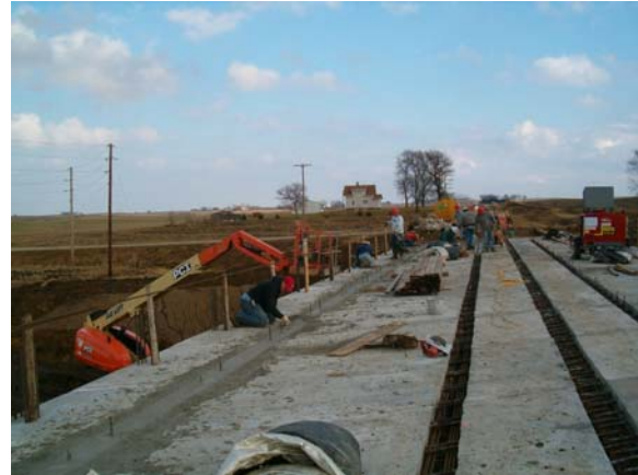
Figure 45 – Casting Long. Joints
