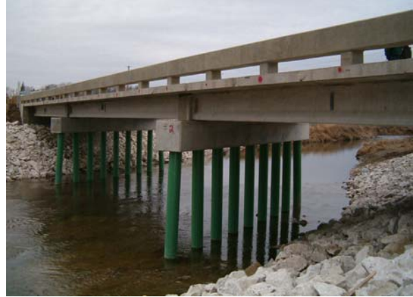
Figure 2 - Completed Mackey Bridge
