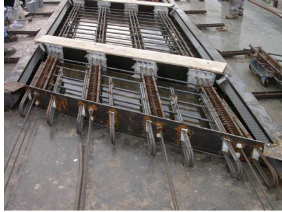
Figure 18 – Longitudinal Joint Reinforcing
