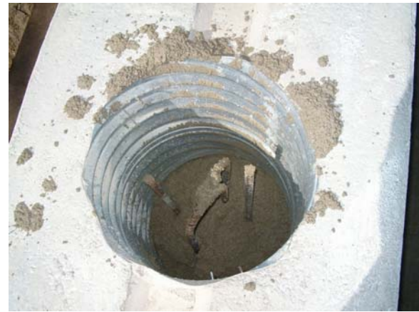
Figure 28 – Filling Pier Blockout
