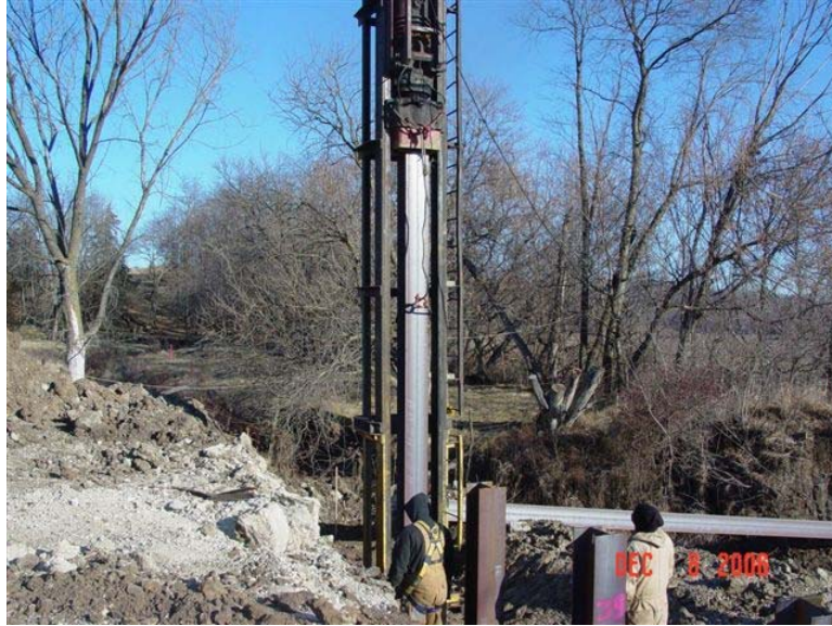
Figure 68 - Driving of steel H-pile at the west abutment
