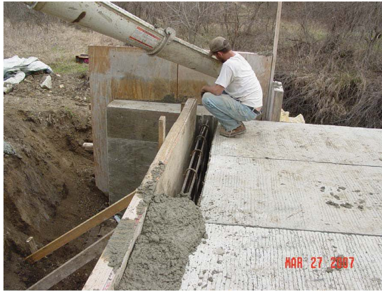
Figure 71 - Contractor placing backwall on the precast abutment
