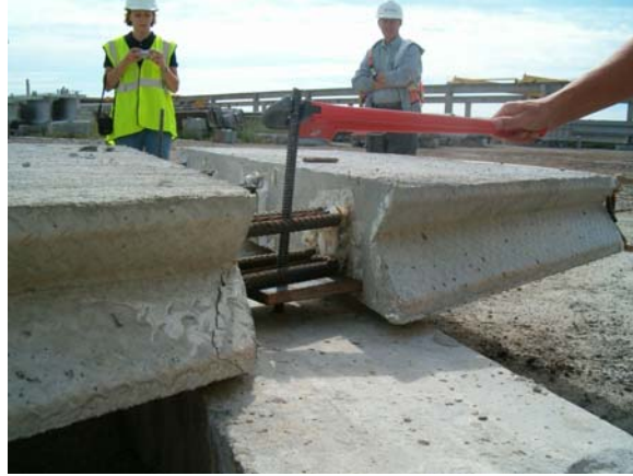
Figure 14 – Leveling Device Test
