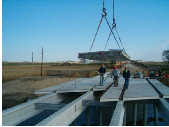
Figure 37 – Deck Panel Erection
