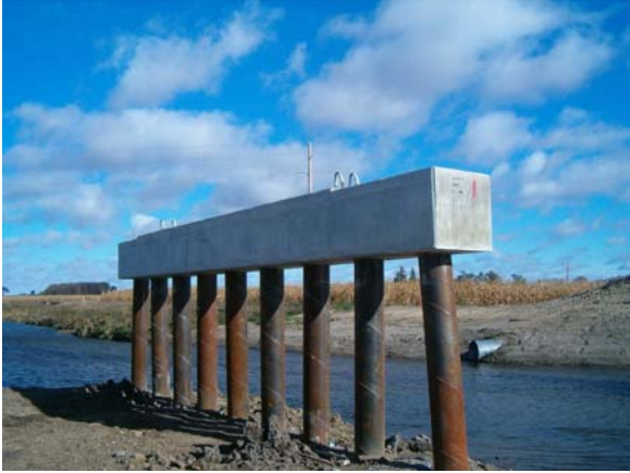
Figure 29 – West Pile Bent
