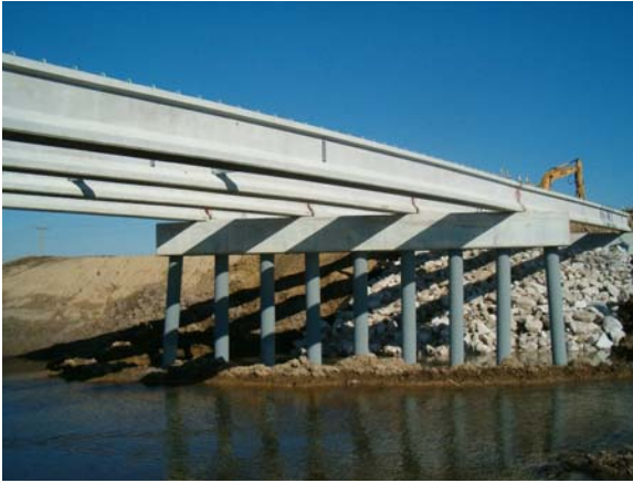
Figure 33 – PPC Beams Erected
