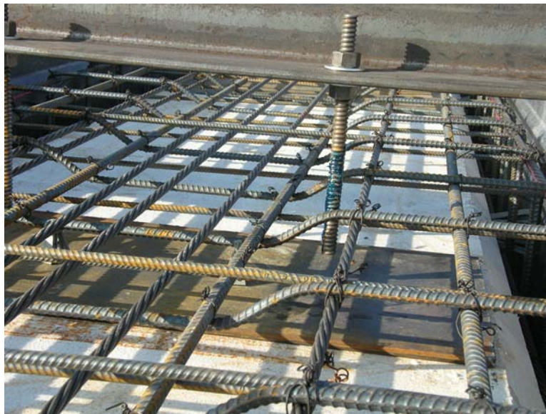
Figure 65 - Detail of Styrofoam insert and hold down system developed by the precaster
