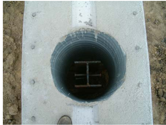
Figure 24 – Abutment CMP Blockout
