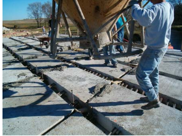
Figure 41 – Casting Transverse Joints
