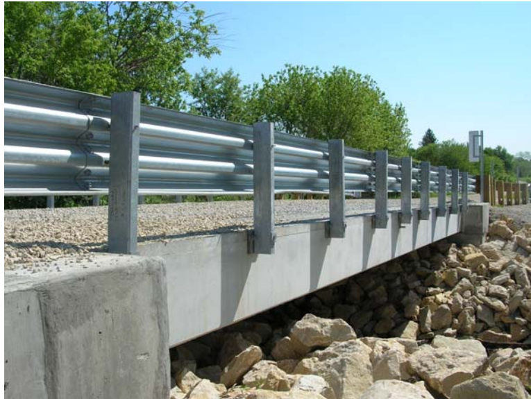
Figure 73 - Profile view of completed bridge
