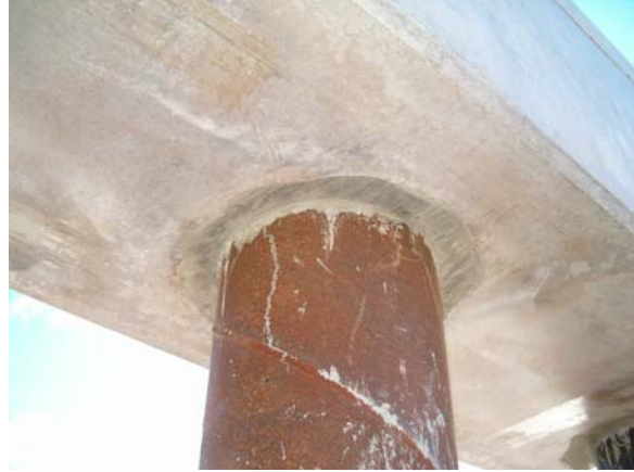
Figure 30 – Pier Cap Connection
