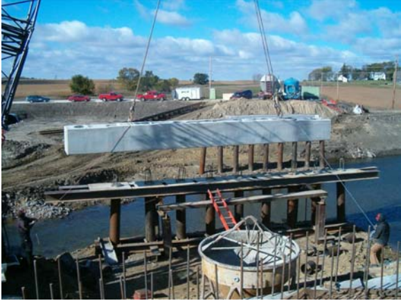
Figure 25 – Setting Precast Pier Cap
