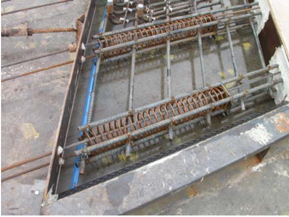
Figure 17 – Spiral Reinforcing
