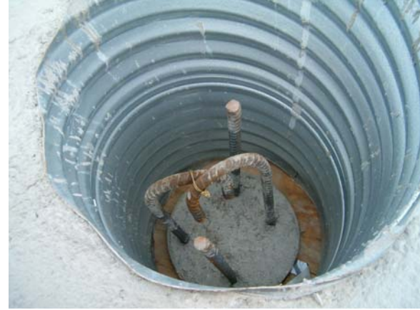
Figure 26 – Pier CMP Blockout
