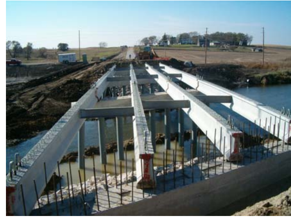
Figure 34 – PPC Beams Erected
