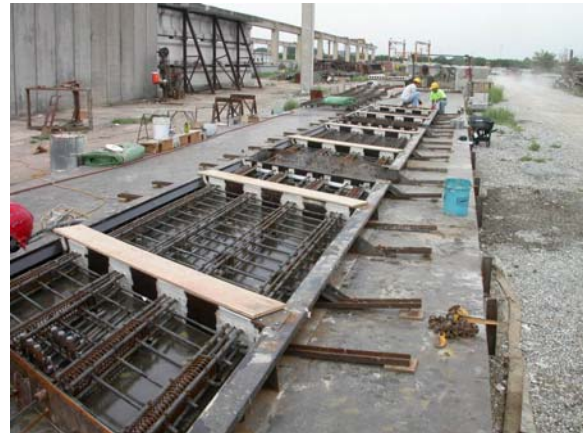
Figure 16 – Panel Form and Reinforcing
