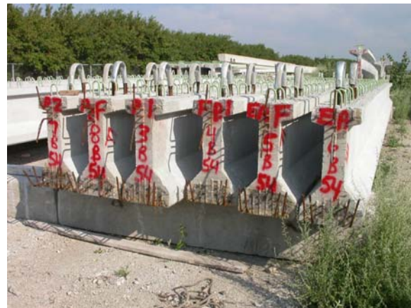
Figure 22 – PPC Beams Stockpiled
