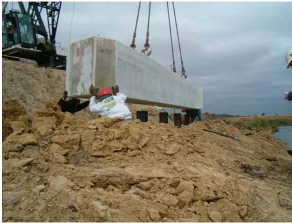
Figure 23 – Setting Precast Abutment
