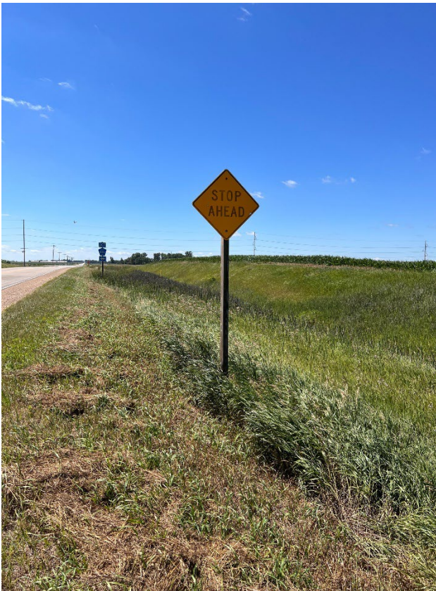
Photo 15. Berm on the east side of the SB approach.
