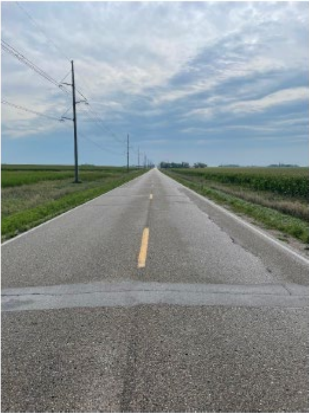
Photo 2. West approach, looking east
