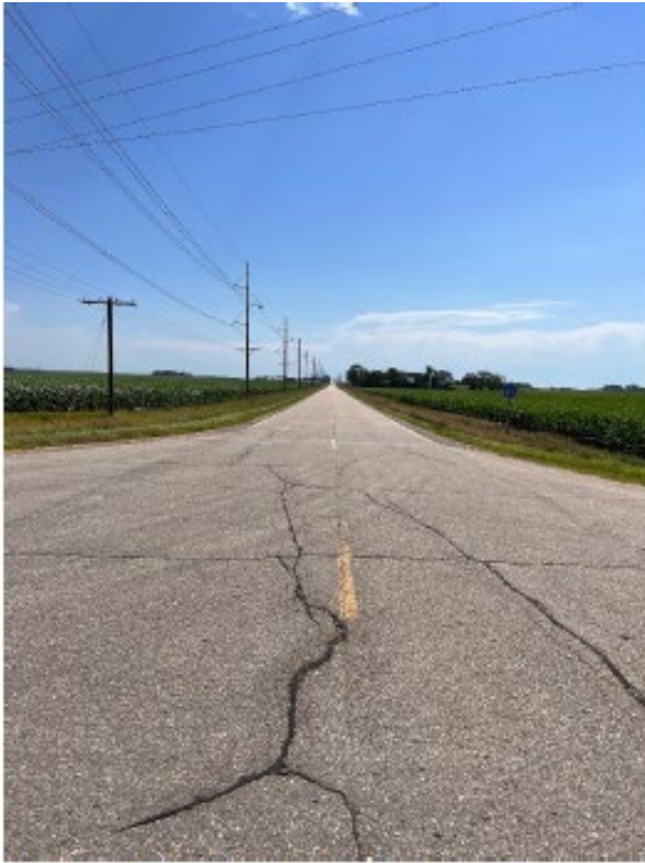
Photo 5. East approach, looking east.
