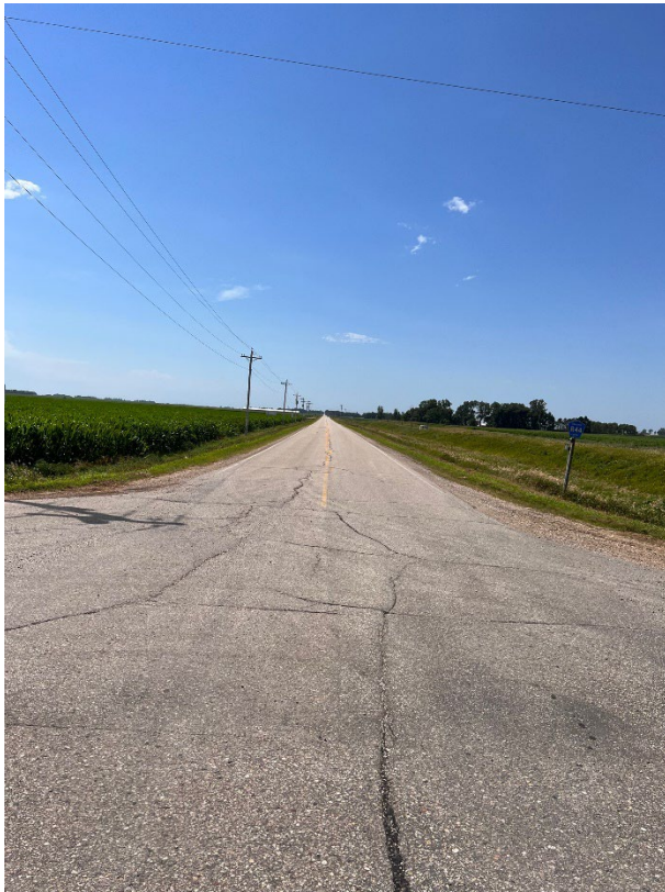
Photo 3. South approach, looking south.
