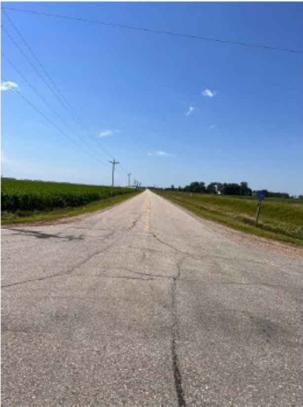
Photo 3. South approach, looking south.
