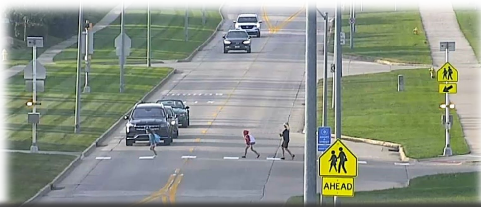
Students using a recently installed RRFB on their way to school in West Des Moines
