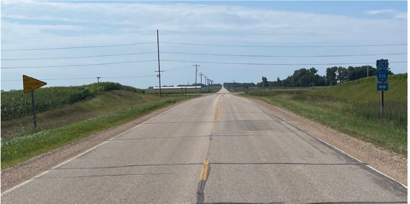
North leg looking South (Expanded View)
