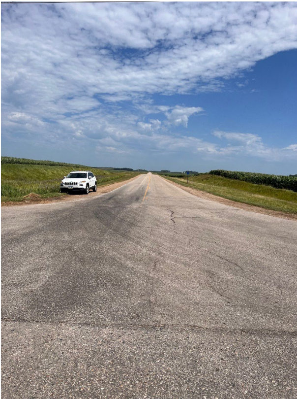
Photo 7. North approach, looking north.
