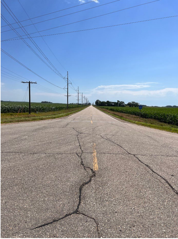
Photo 5. East approach, looking east.
