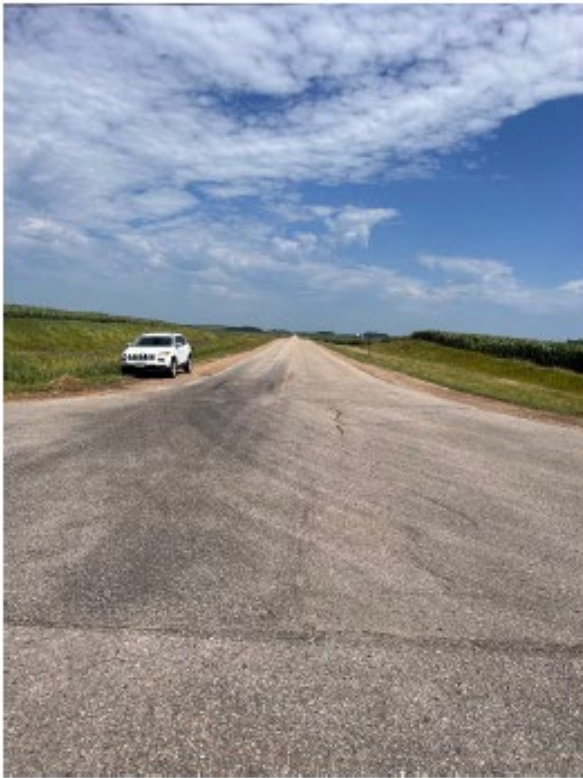
Photo 7. North approach, looking north.
