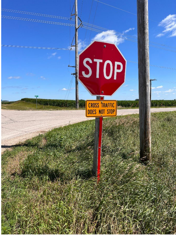
Photo 9. Damaged NB stop sign.
