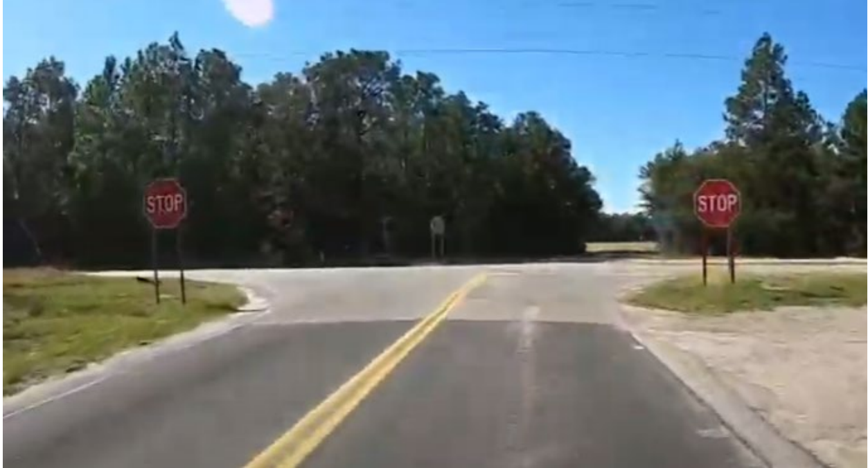
Photo 16. Oversize STOP signs on the right and left and no passing zone markings on approach.
