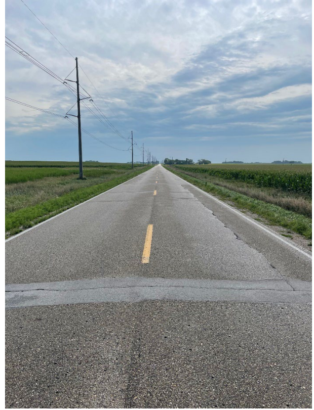
Photo 2. West approach, looking east
