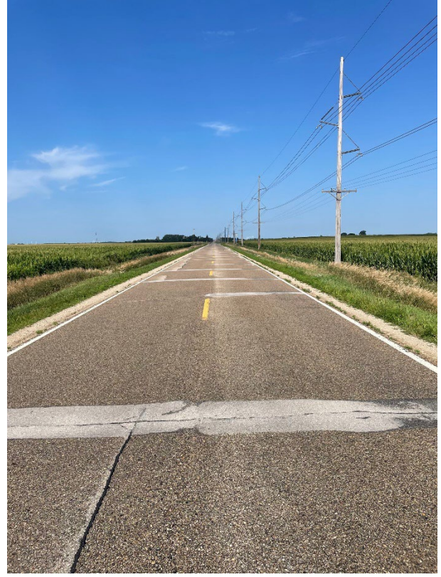
Photo 6. East approach, looking west.
