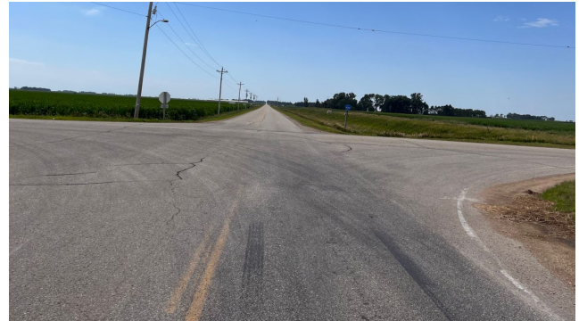
Photo 14. Stop Line for SB stop condition.
