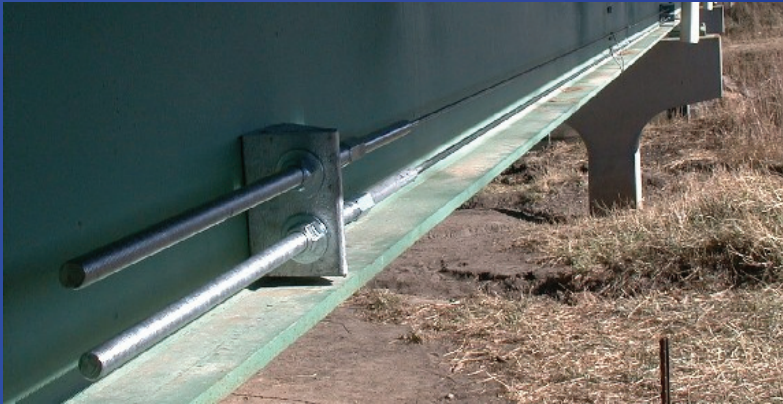
End Span (Exterior)
